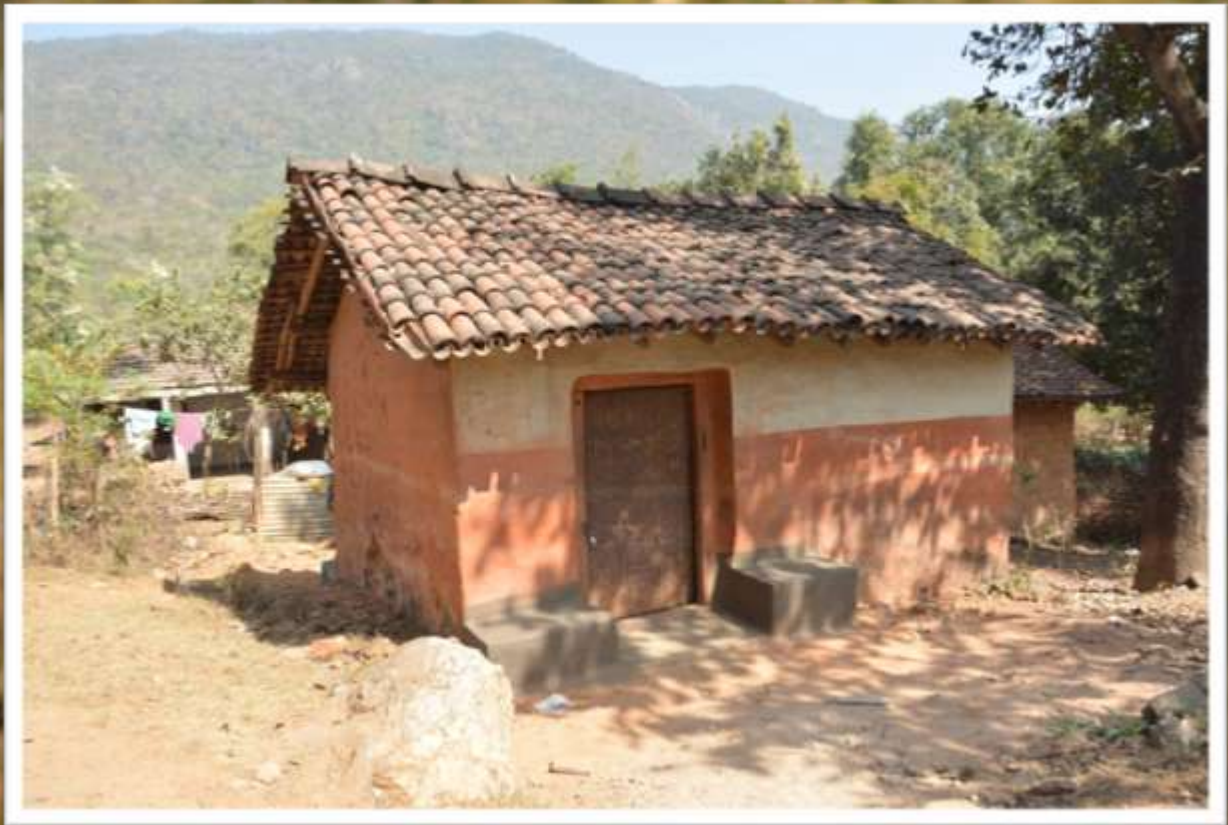
Pic-1.Front view of the house, Place- Pattipani, Jharkhand.Date-02.02.14 Serial No.1 (a), Cf.. 2
