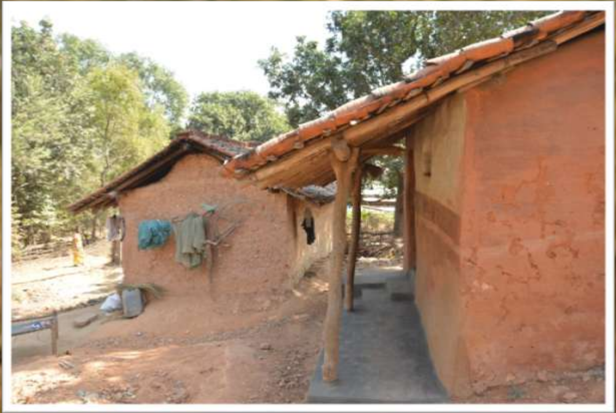
Pic-4. Side view of the house. 'hasa oṛa' Pattepani. Date-13.02.14. Serial No. 1(c)
