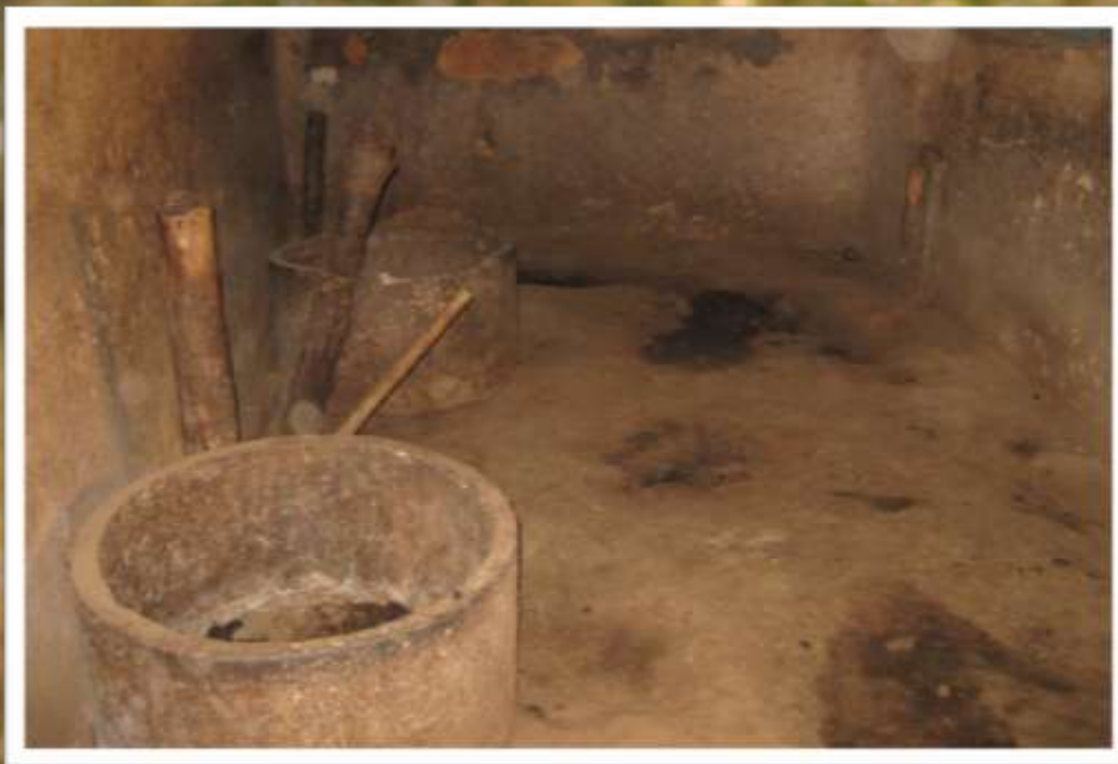
Pic-11. Interior view of Cowshed. Bhadua. Date-13.02.14. Serial No. 1(e)
