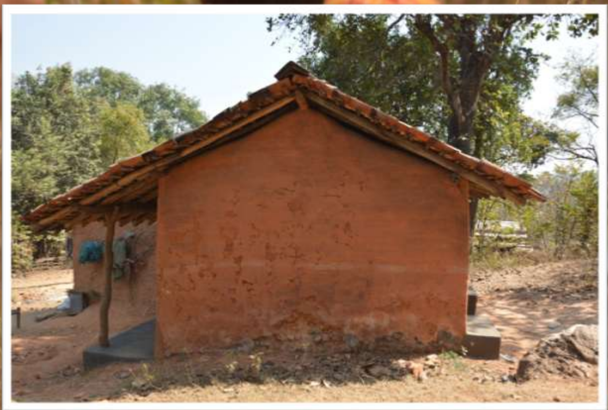
Pic-3.Side view of the house. 'hasa oṛa' Place- Pattepani. Date-02.02.14. Serial No. 1(c)
