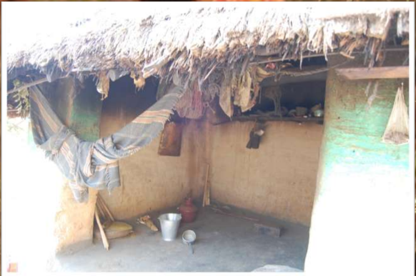
Pic-1(a). Front view of the house, Place- Bhadua. Date- 13.02.14. Serial No. 1
